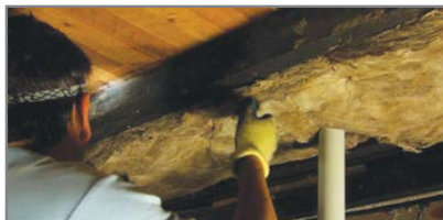
Cutting insulation to install around plumbing services
