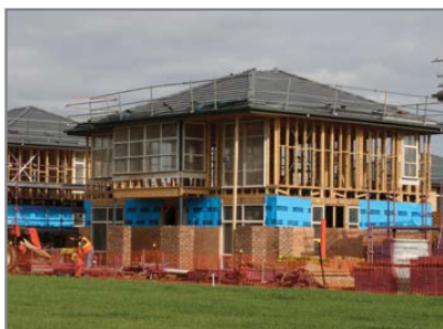
Safety rails fitted for working at heights
