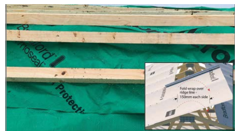
Install sarking from gutter to ridge
