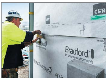
Taping and sealing membrane overlaps
