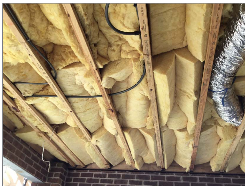
Batts squashed into rafters compromise thermal benefits
