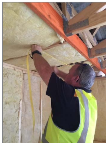
Installing ceiling batts with stringing in method.
