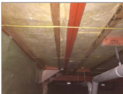
Stringing under floor insulation in place
