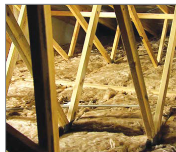
Fully installed ceiling insulation batts - no gaps
