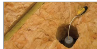
Check table minimum clearances for recessed lumen.
