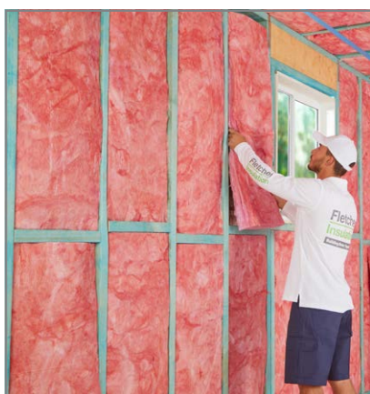
Examples of well installed wall batts
