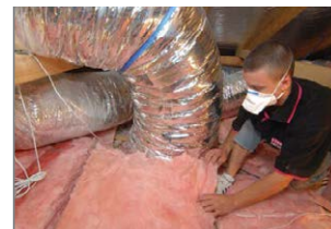
Fitting insulation snugly around ducting
