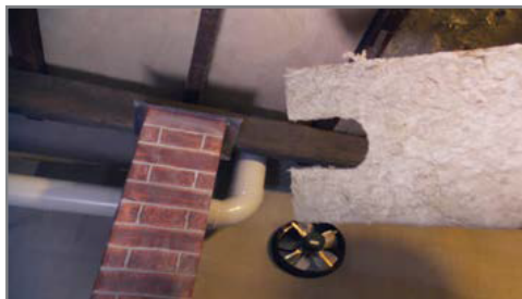
Cutting insulation around under floor services
