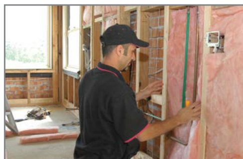
Installing insulation behind services
