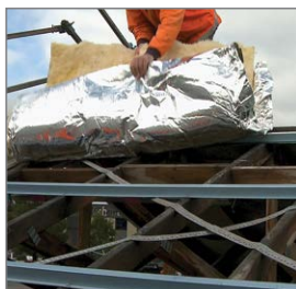
Vertical roll out over horizontal battens
