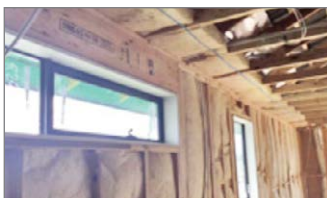
Installing perimeter batts over top plate
