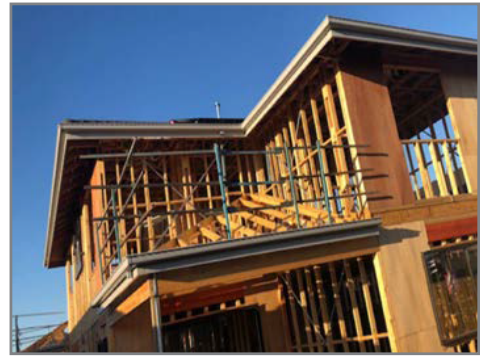
Roof edge fall protection.
