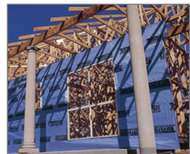
Fixing wall wrap neatly around windows
