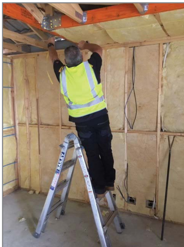
Example of fitting edge batts
