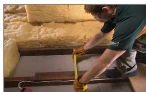
Measure - right sized batts
