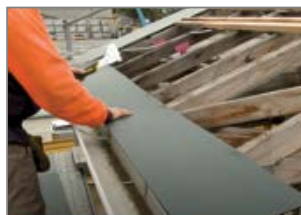
Fixing anti-ponding board
