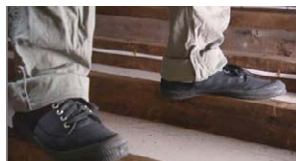
Safety: use joists for footing support
