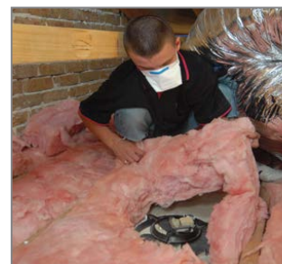
Check table minimum clearances for recessed lumen.
