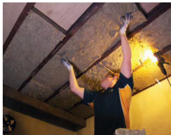
Elevated floor- installing insulation between floor joists
