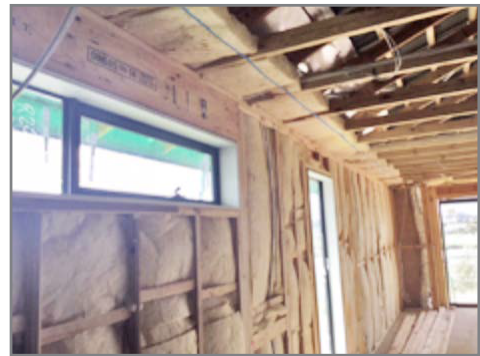
New build - perimeter batts installed.
