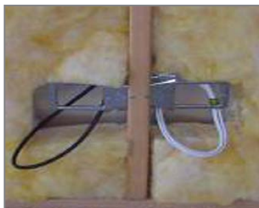
Insulation cut-outs for power points
